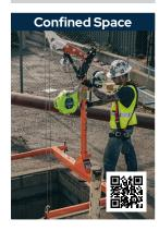
Commonly used to raise and lower personnel in confined work spaces, davit and tripod systems are essential components of any confined space entry and retrieval plan.
